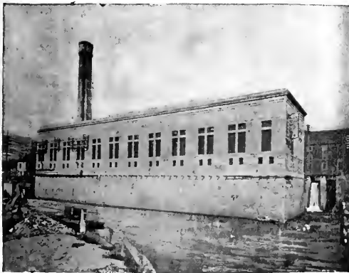
FIG. 3.—EXTERIOR VIEW OF HYDRAULIC POWER HOUSE.
